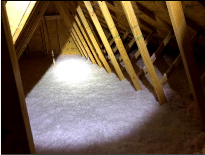
Attic - Insulation sample photo
