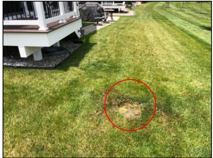
Ponding water, sample
