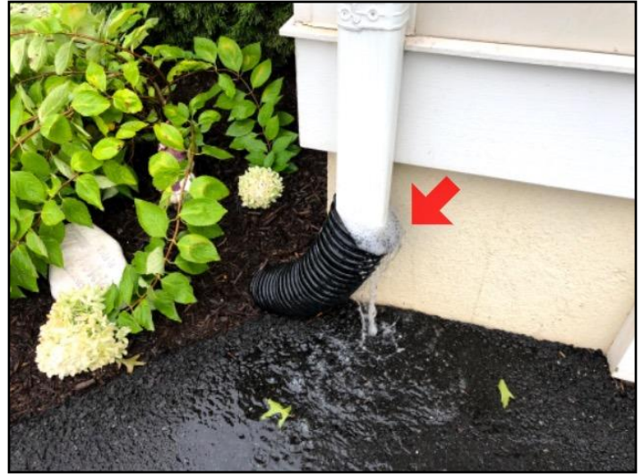
Not properly connected. Repair Recommended
