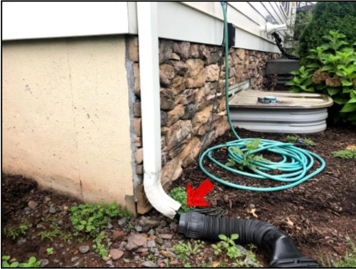
Not properly connected. Repair Recommended
