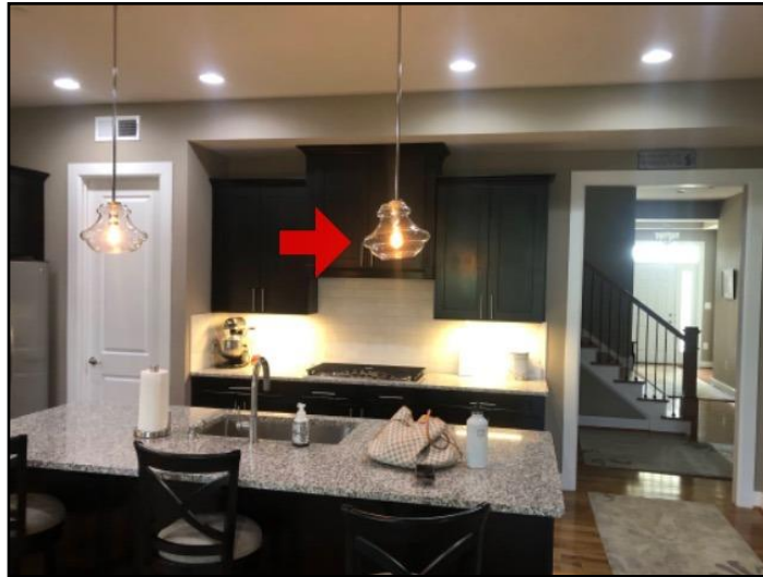
Lighting fixture is slightly cockeyed
