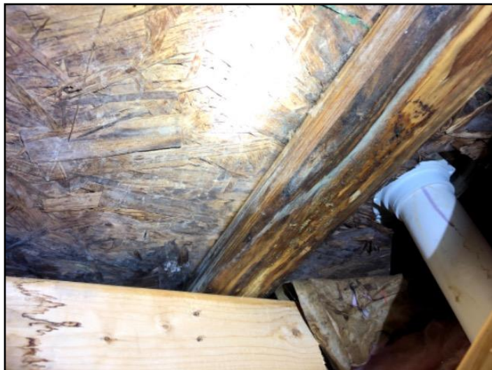
Primary Bathroom OSB Subfloor, sample
