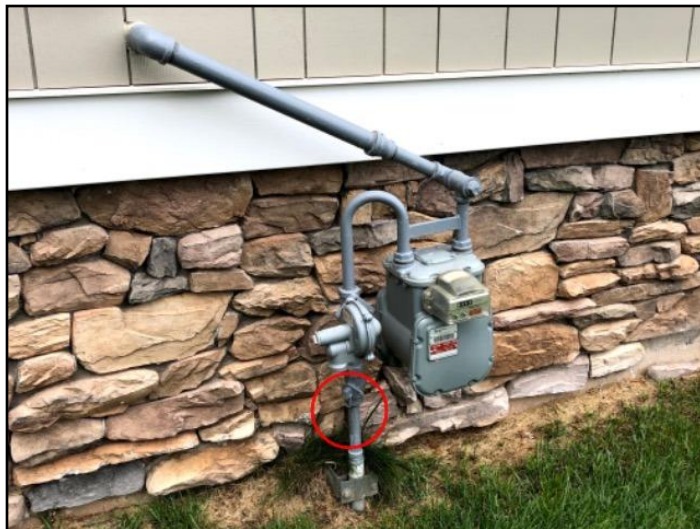
Main gas shut off valve
