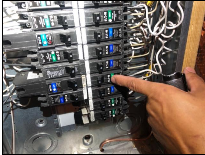
(AFCI) test faulty, sample
