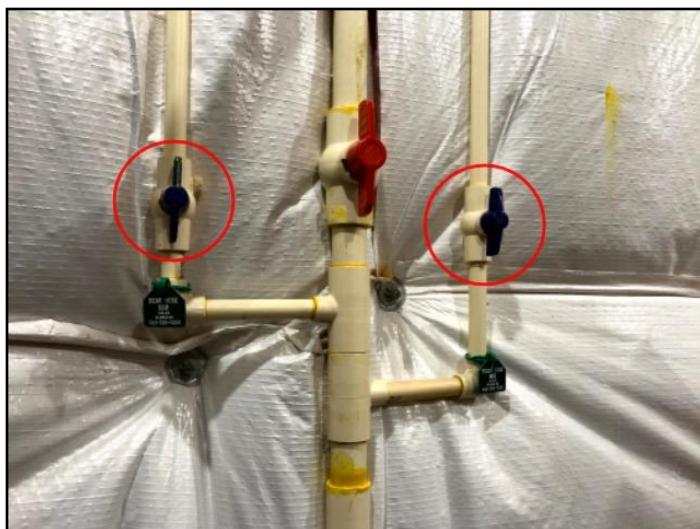
Exterior hose bibb - shut off valves
