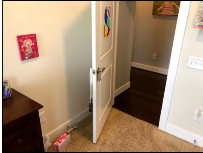
Does not latch properly
