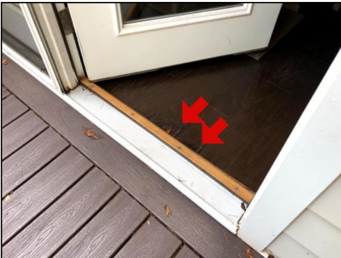
Evidence of leakage - Locatioin sample photo
