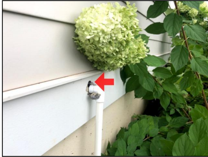
Penetrations should be sealed, sample
