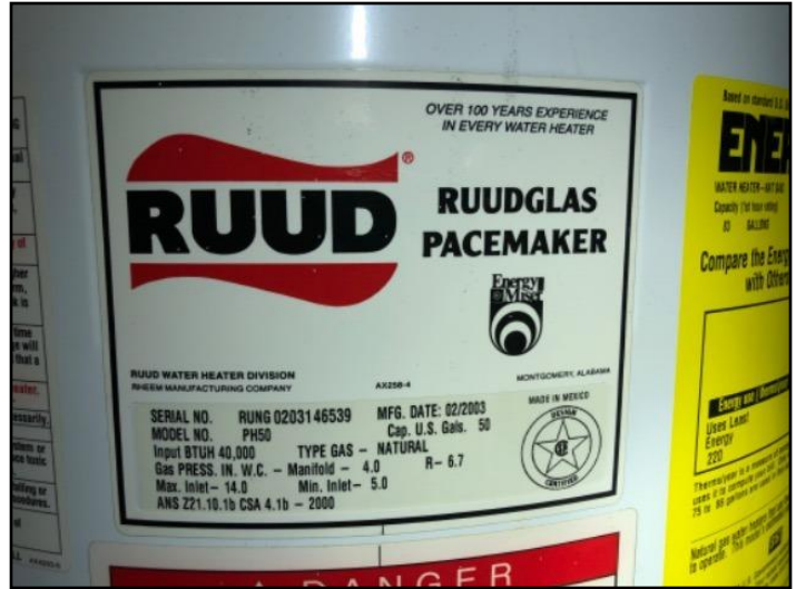
(2003) Water heater data tag sample
