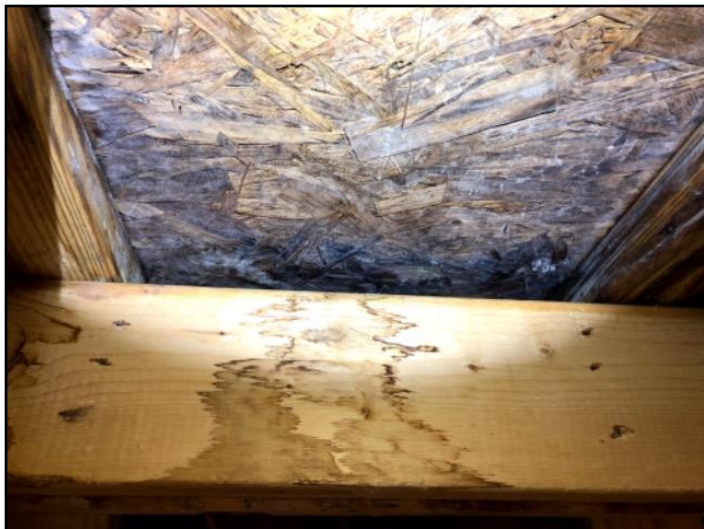
Primary Bathroom OSB Subfloor, sample
